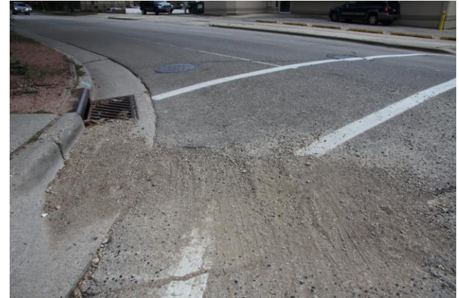
Erosion and vehicle tracking from construction sites.
