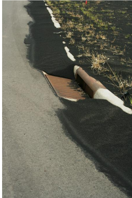
Erosion and vehicle tracking from construction sites.
